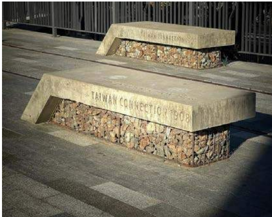
Precast concrete / gabion stone baskets
