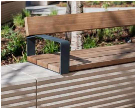
Timber / steel seating
