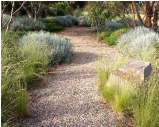
Compacted rubble / stabilised fines
