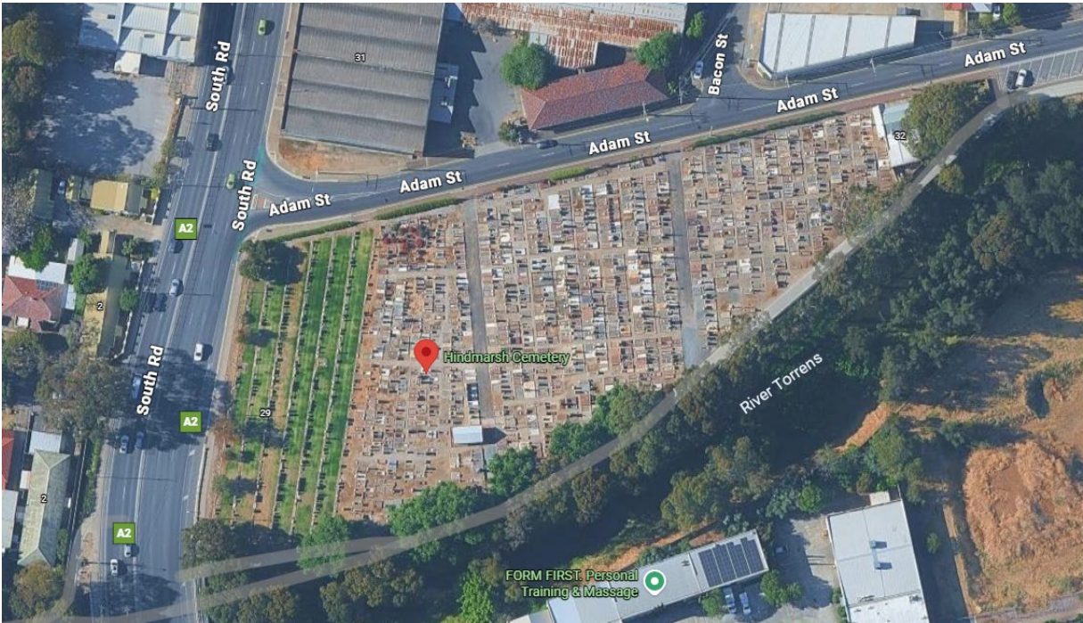
Figure 01: Aerial image showing extent of Hindmarsh Cemetery.
